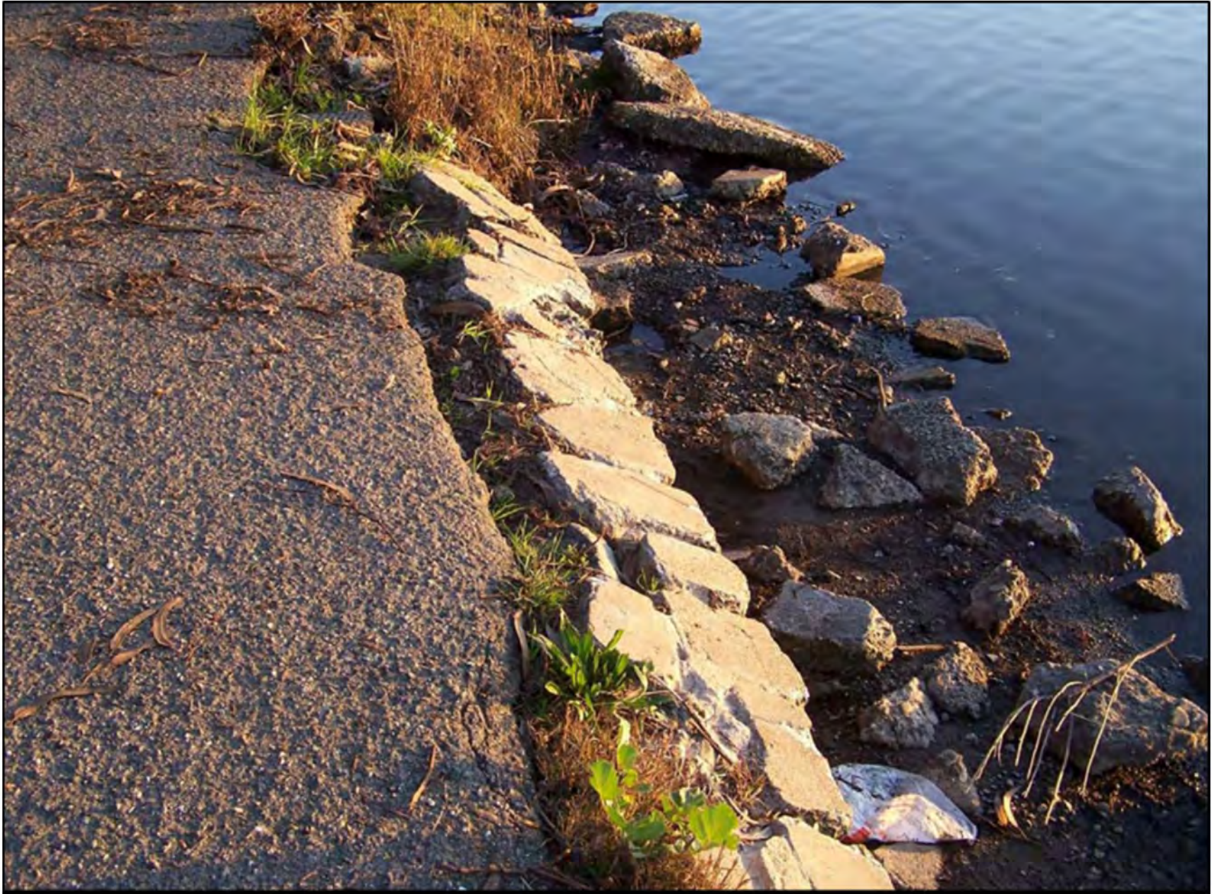
Figure 53: Rock Wall Falling off Shoreline Trail on East Shore of Main Lagoon
