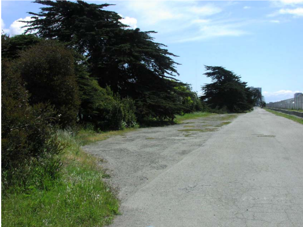
Figure 3-43. Western Shoreline Abandoned Parking Lot #3
