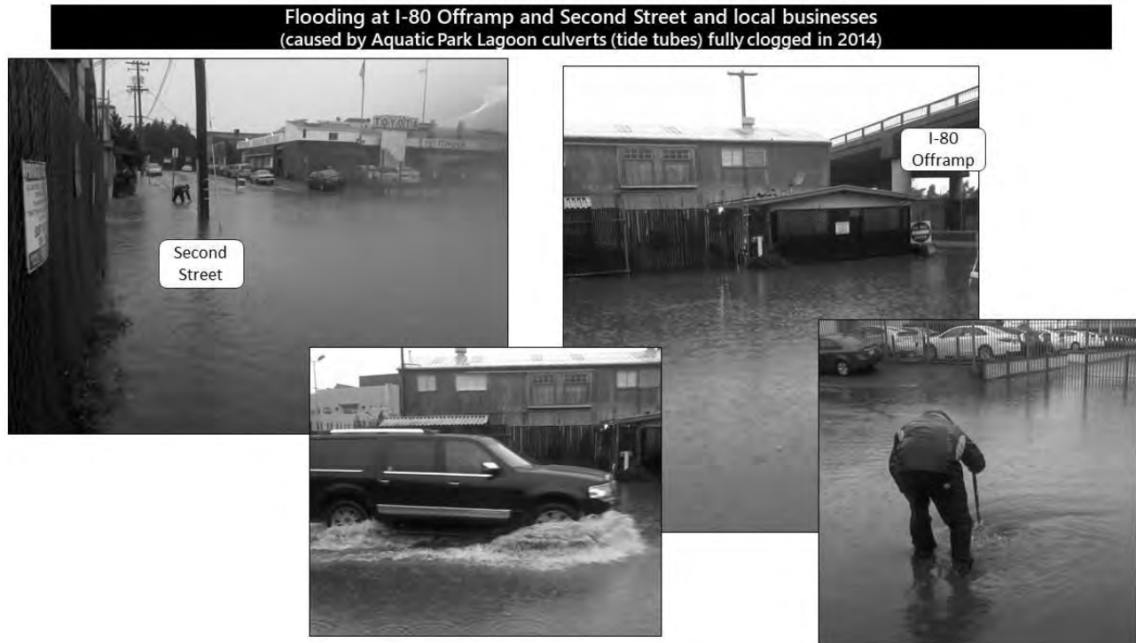
Figure 4: I-80 Offramp and 2 nd Street Flooding
