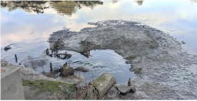
Middle lagoon at low tide. Above, inflow comes from lower pipe largely blocked by sediment. Note location of ripples. Upper pipe, shown by arrow at right, is broken and non-functional.
