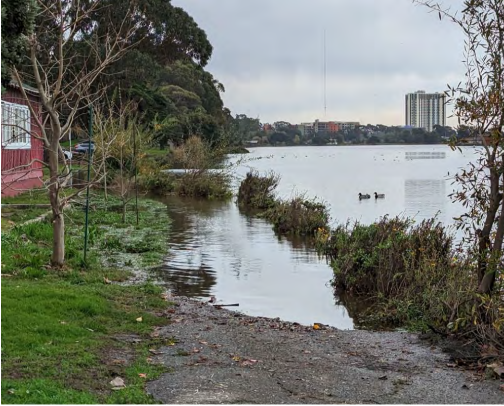
Due to extensive rains, the water level rose and blocked the walking pathway, extending into the parking lot. Jan 2023
